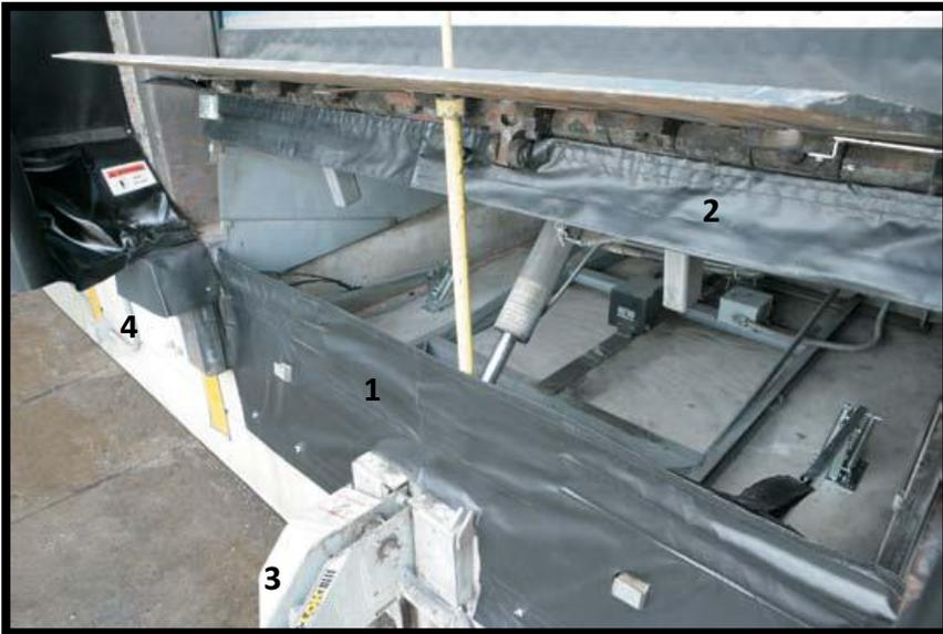
1. The main sealing curtain made of durable black vinyl is held in place by spring-loaded pivot arms and flexible stays that keep the seal engaged against the leveler and pit sides.
