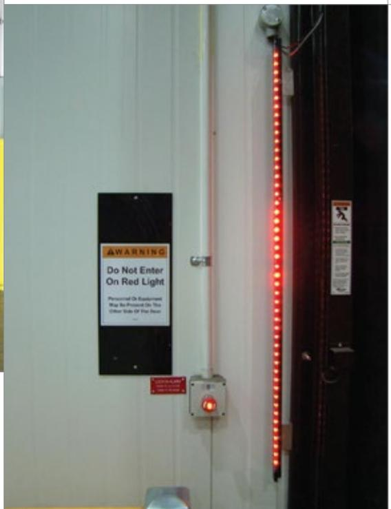
Collisions between forklifts and pedestrians are the second most common type of forklift accident. Our Advanced Warning Technology helps reduce these dangerous and costly mishaps. This safety light communication package uses motion sensors and LED lights to alert forklift drivers to people, objects or equipment moving on the opposite side of a closed door, door opening, blind corner, or facility intersection.
